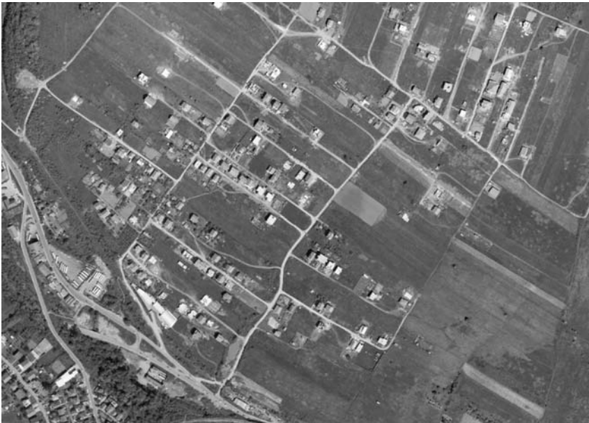
Figure 4. Areal photo of part of Jelezovac informal settlement (Source Republic geodetic authority of Serbia).
