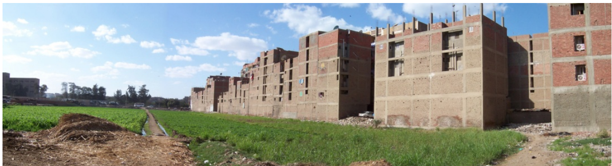
Figure 5. Bulaq al-Dakrur. A non-built sector let see the typical concrete skeleton on the buildings' backside. Source: Authors, 2006.
