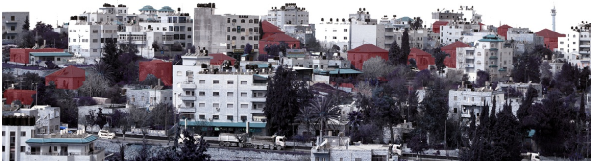
Figure 3. Old Centre of Ramallah - a panorama image differentiating old structures from new. (source: author)
