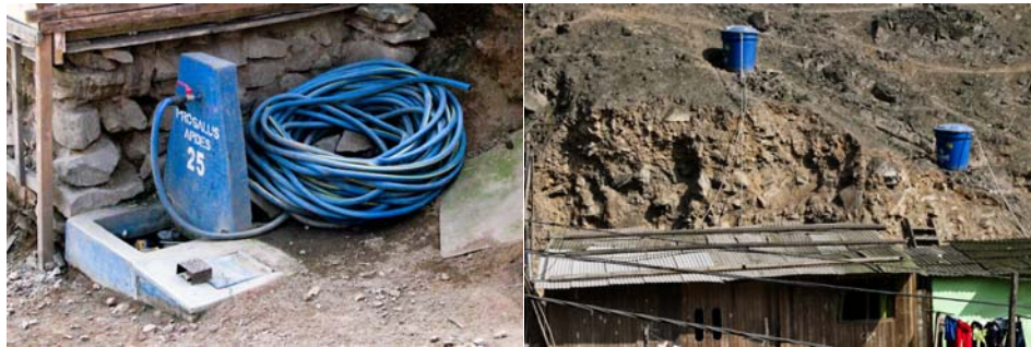
Figure 2: Progressive water system from community standpipe to individual tankers through hoses (Settlement Señor Cautivo de Ayabaca, District of Comas, photos by the author, 29/08/2012).
