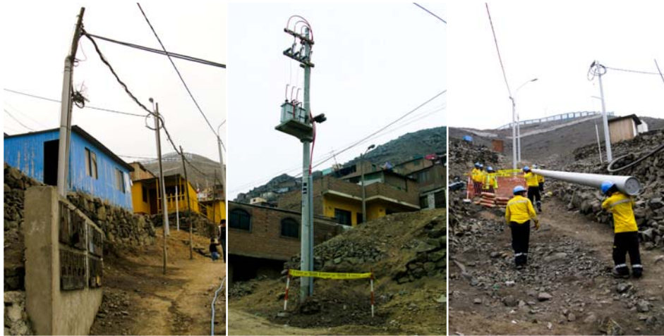
Figure 1. Innovations for electrification: Macro-meter and wooden provisional posts, Single-post transformer yet to be connected, Installation of fibreglass post (Settlement Año Nuevo , District of Comas, photos by the author, 16/08/2012).
