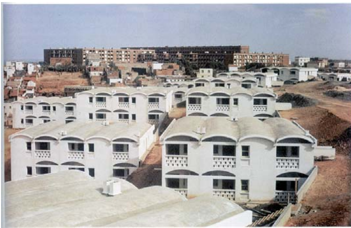
A_ Kopp, P_ Chazanoff, Rehabilitation de Oued uchaia 1963-65
